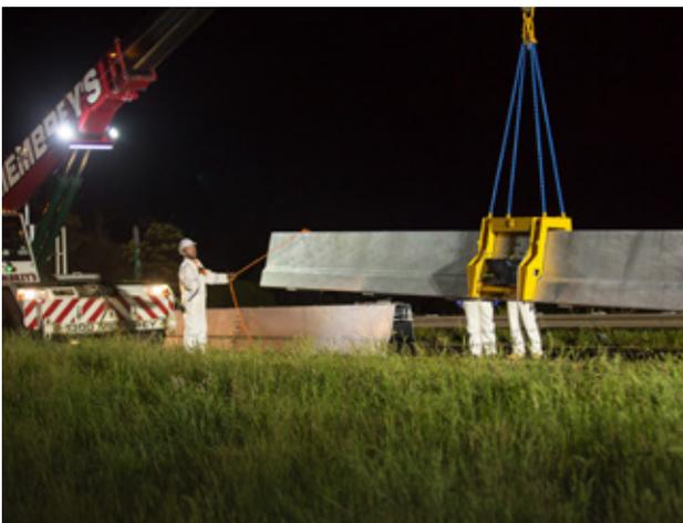
Barrier being installed to the median area of the Monash Freeway sections from EastLink to Clyde Road to create work zone for workers.
