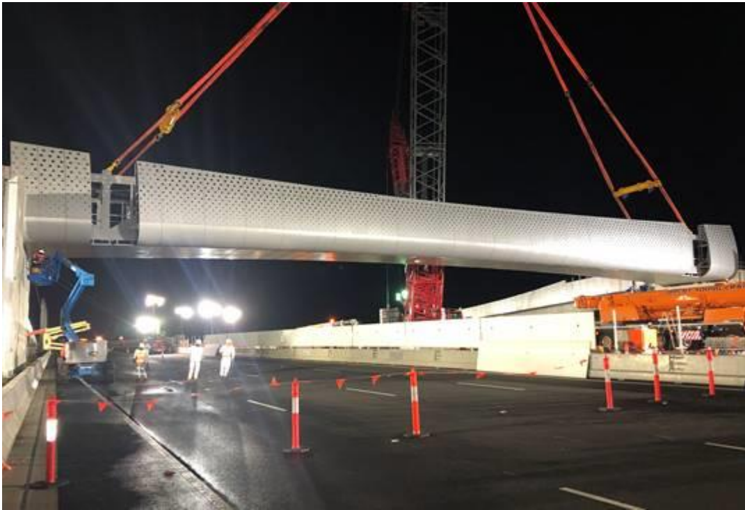
Rosala Avenue overpass is safely positioned across the West Gate Freeway.
